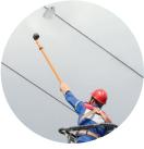
Installation on the line without disconnecting the voltage – using a simple hot stick tool
