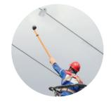
Lodestar CL4 BM is mounted on the overhead phase conductor. The live-line installation is possible using a standard hotstick tool
